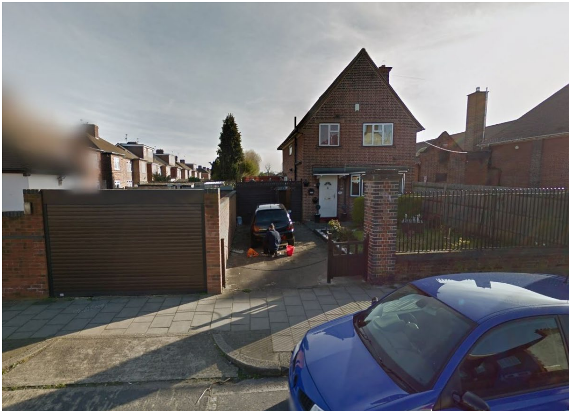
Photo 1 – Front elevation of property.
